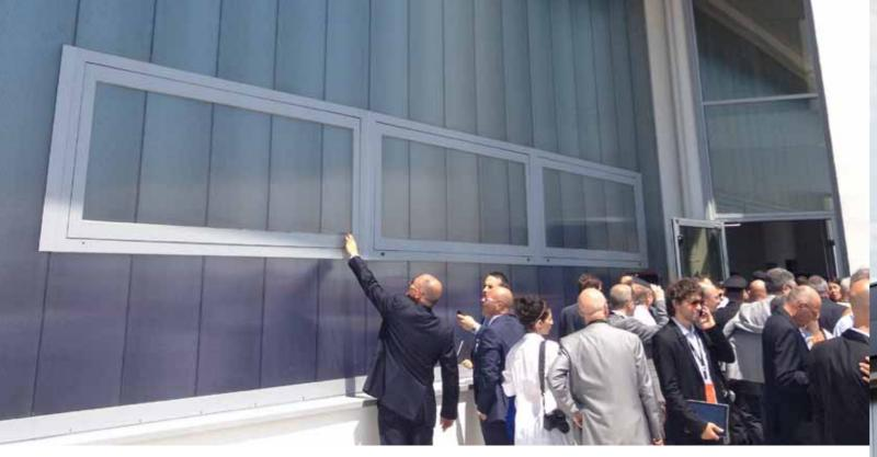
The function of the IR treatment is to absorb the infrared component of solar radiation (780 to 1400nm), blocking solar radiation responsible for the greenhouse effect, while permitting the passage of the visible component.
